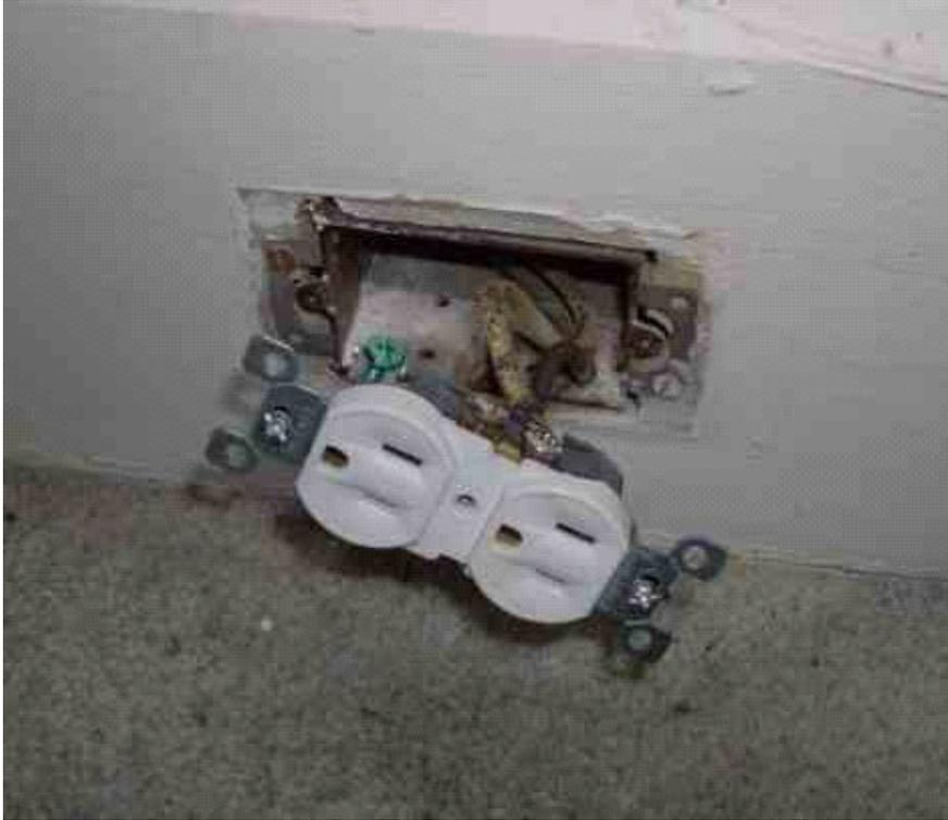
*Here a 3-prong outlet was used to replace on older 2-prong outlet in a 2-wire, ungrounded system. (The metal box here is not grounded.)*
